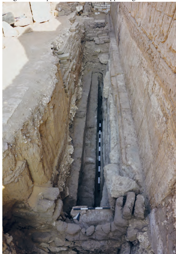
Fig. 12: M3, retaining wall 13-18-191
